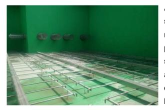
A stainless steel coarse bubble aeration system is employed to mix the suspended media evenly throughout the reactor while providing the mixing energy required to slough old biofilm from the internal surface area of the media and maintain the dissolved oxygen required to support the biological treatment process.
