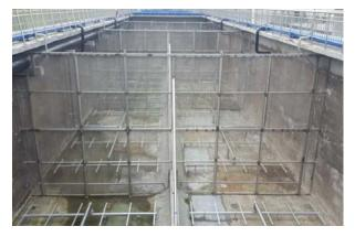
limits the treatment capacity of activated sludge systems. IFAS technology addresses the need for increasing activated sludge plant capacity without additional clarifier or aeration basin volume. The fixed biomass also contributes to the ability of the process to respond to organic or hydraulic shock loads and to recover from upsets.
